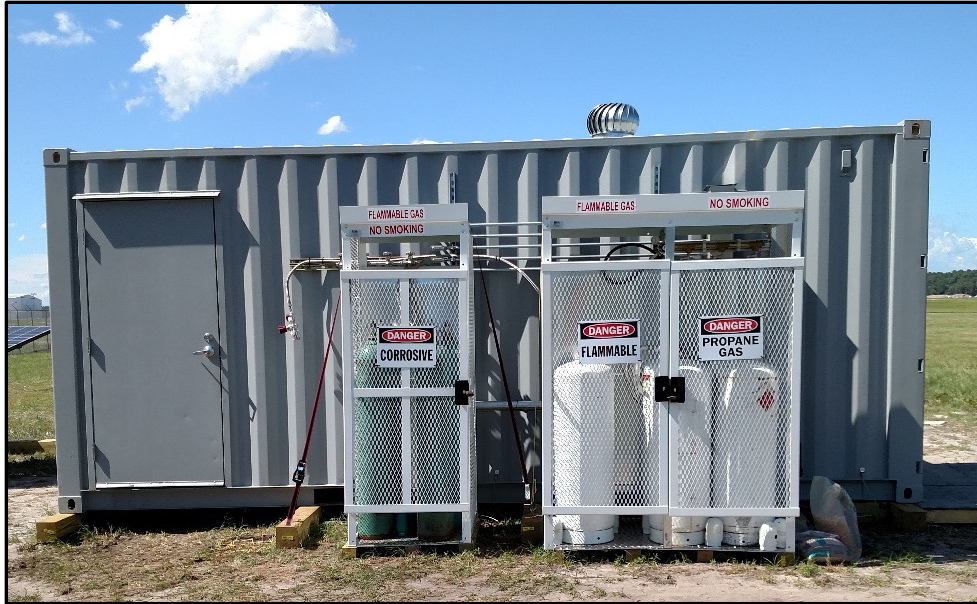
Figure 5.24. Photograph of Propane and Ammonia Gas Storage.
