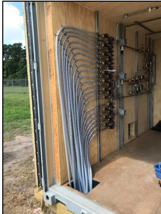
Figure 5.23. Photograph of Tubing Connections to the Biosparging System.
