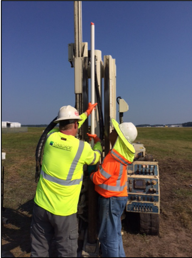
Figure 5.13. Photograph of a Direct-Push Well Installation.
