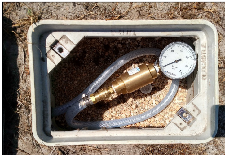
Figure 5.21. Photograph of Biosparging Well Head Assembly.
