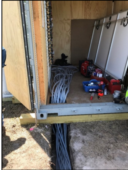
Figure 5.22. Photograph of Gas Tubing Installation.
