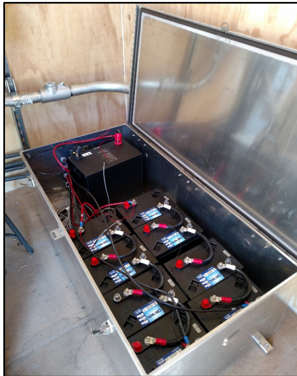
Figure 5.27. Photograph of the 24V and 48V Solar Power Battery Systems.
